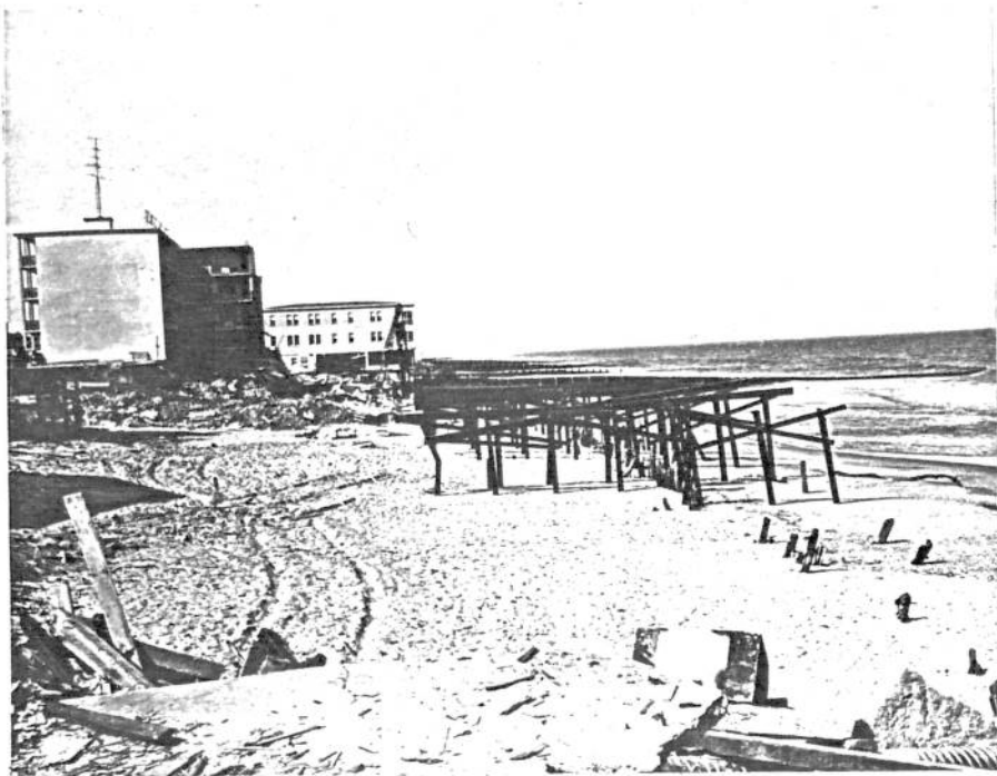
Figure 3. Photograph of property damage at Rehoboth Beach, Del. following the March 1962 storm.
